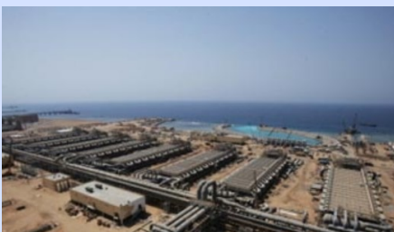
Shuwaikh Seawater Desalination Plant, Kuwait City Fuente: MENAFM
