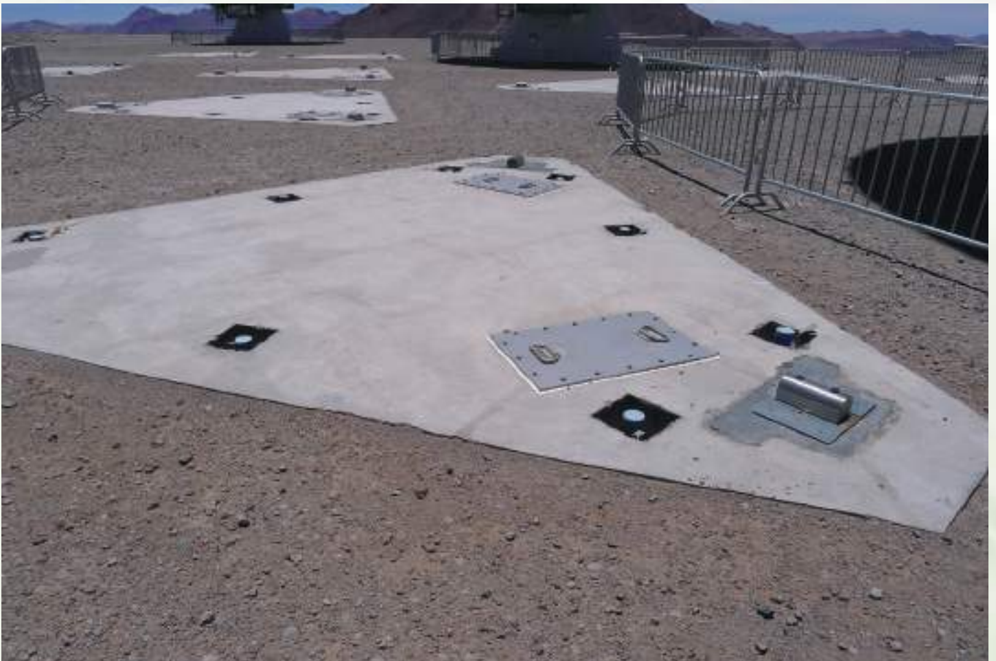
[ESO] Ridge Interface plates for the foundation of antennas for the Atacama Large Millimeter Array (ALMA), 2010
