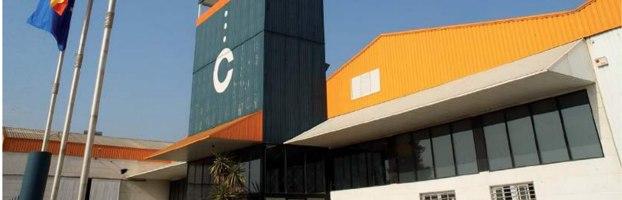
Fachada principal de IMECAL, S.A.
