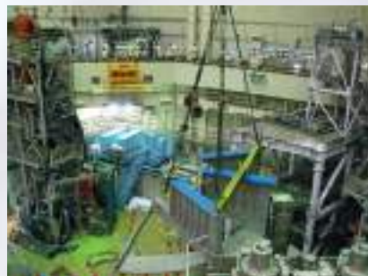
Assembly of Cryostat Base
