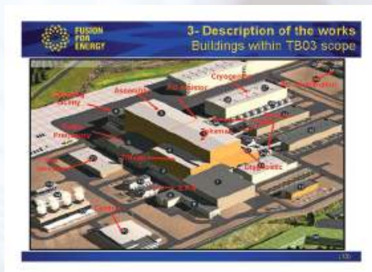
TB03 – Main Civil & Finishing Works
