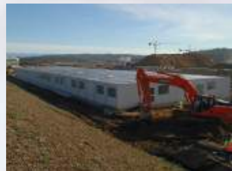
Site Adaptation Works: canteen
