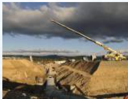
Site Adaptation Works: trenches
