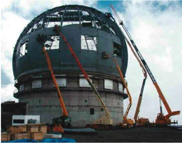
GRANTECAN dome erection
