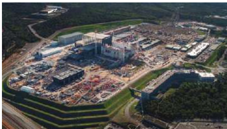
Aerial View_October 19_© ITER Organization-EJF Riche
