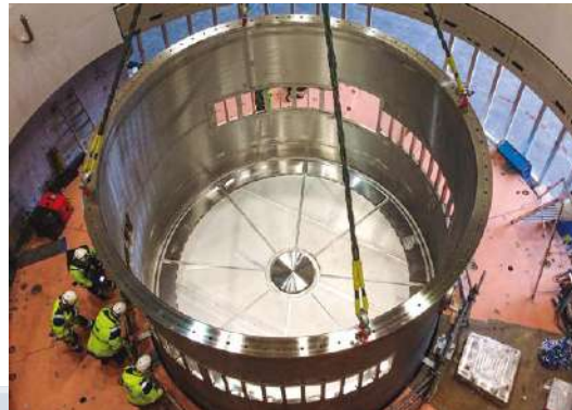
Monolith Vessel Installed in ESS ERIC
