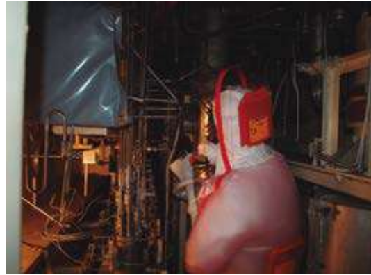
Nuclear Decontamination at CIEMAT
