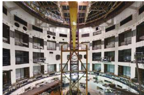
Tokamak Assembly pit_March 19_© ITER Organization-EJF Riche
