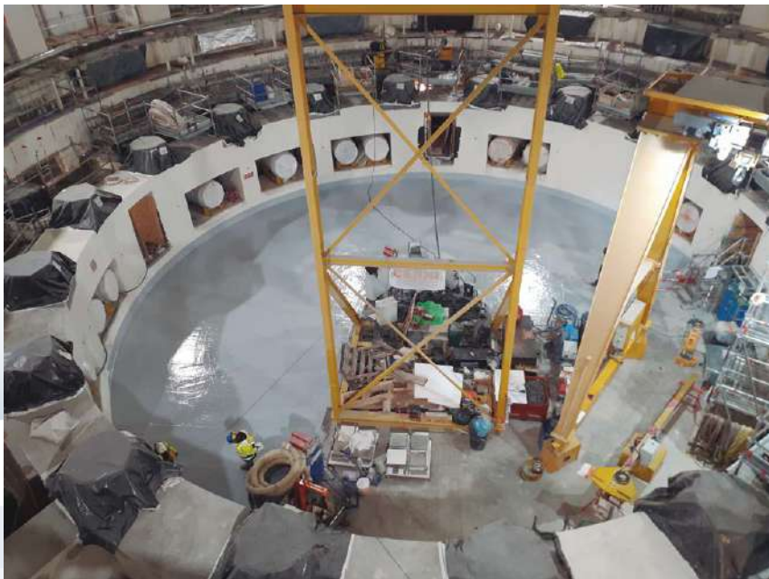
GDES Revanti - Tokamak Building- ITER
