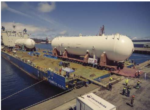
Transport and load out of 5 Slug catchers of 2000 tons in Gijón
