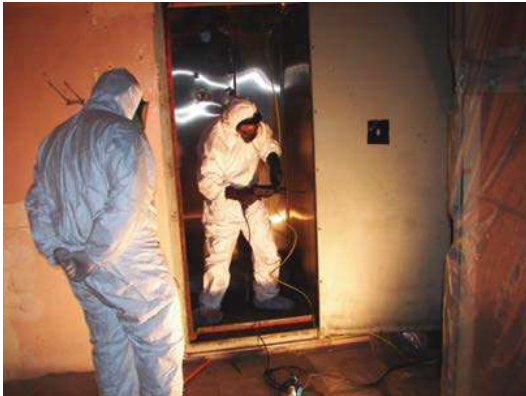
Nuclear Dismantling works
