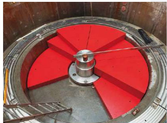
ESS - Vessel support and Ground Shielding
