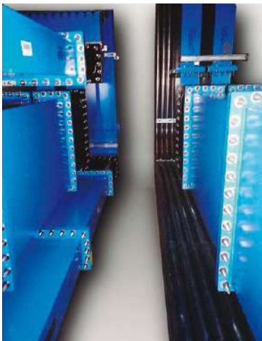
ESS ERIC RF Transmission Line Installation
