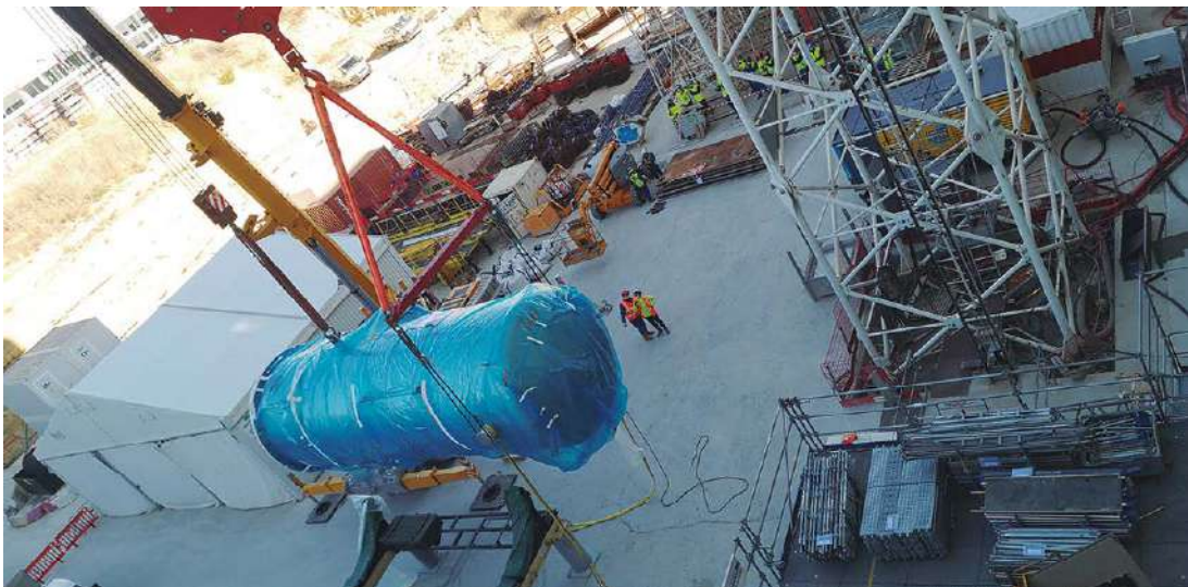
Vessel Installation at ITER
