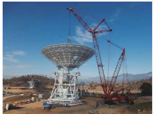
DSN 34m antenna installation in Australia
