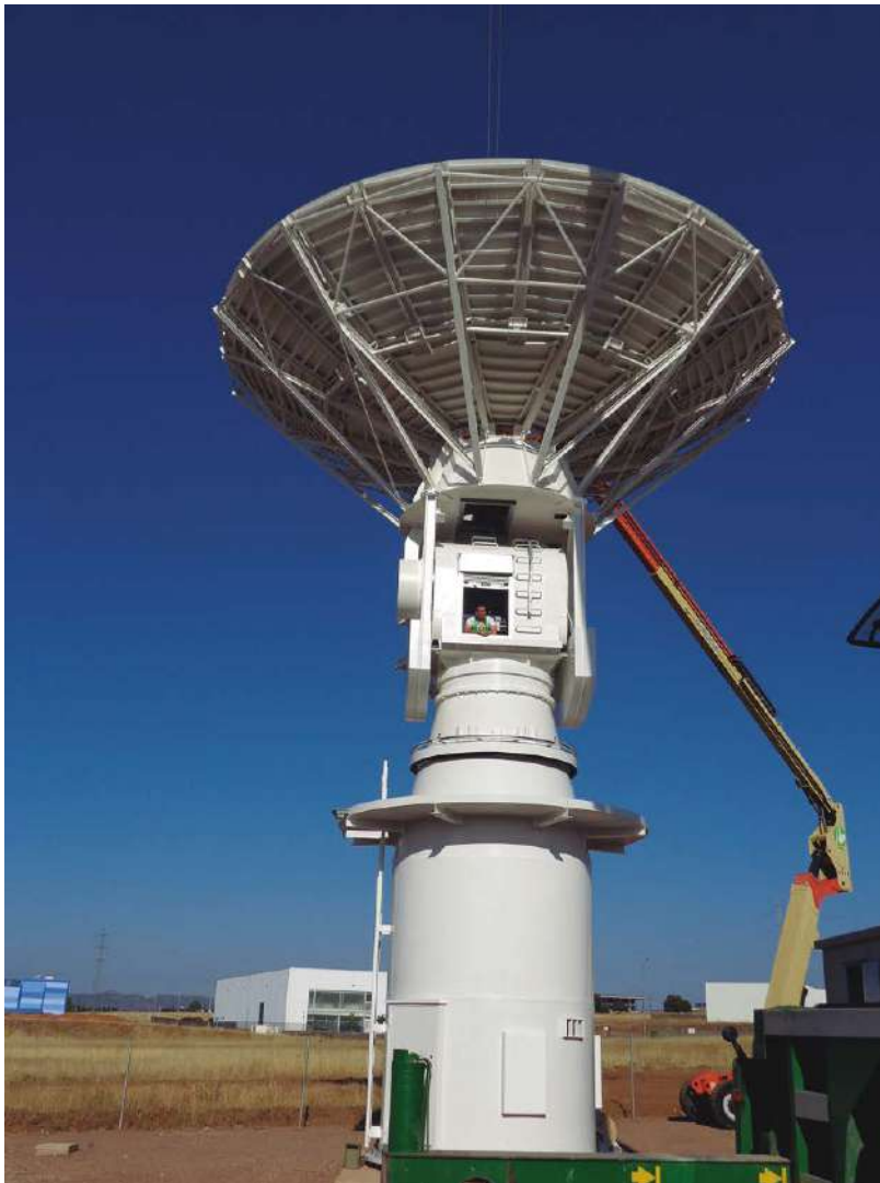
Deimos Ground Station - Elecnor Deimos - Integration of the 10 m TTC Ground Station for Deimos-2 Satellite, 2013
