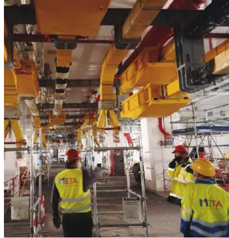
Busbar installation at ITER
