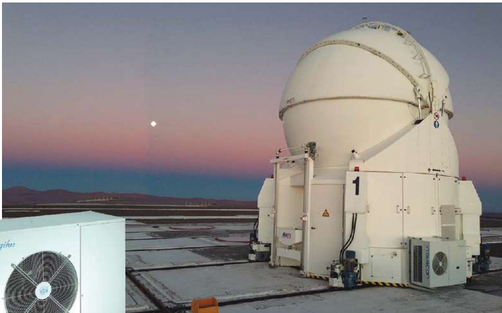
INTARCON chiller installed at ESO premises, Atacama desert, Chile
