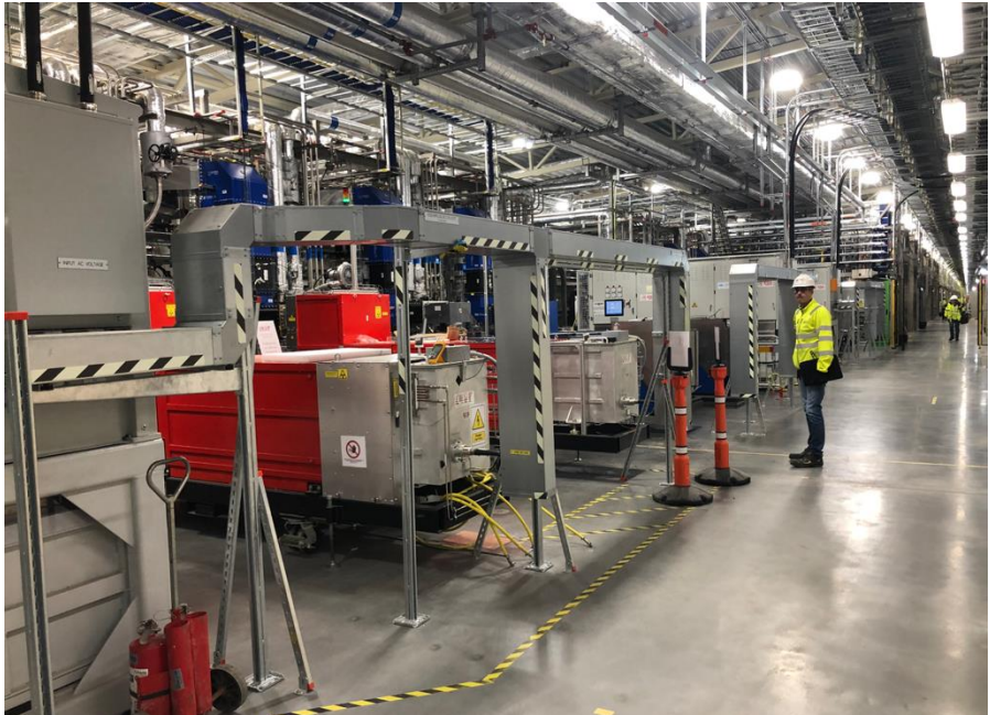
Installation and testing ongoing in superconducting linac
