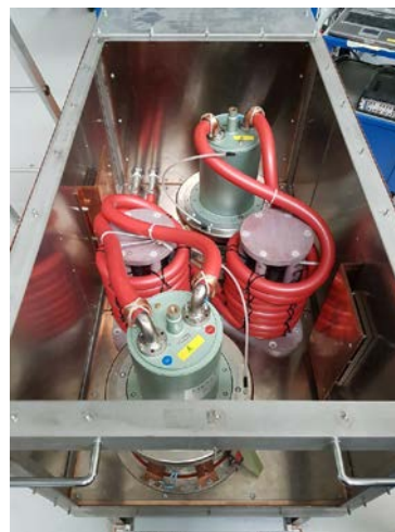
CR debuncher tetrodes (anode)
