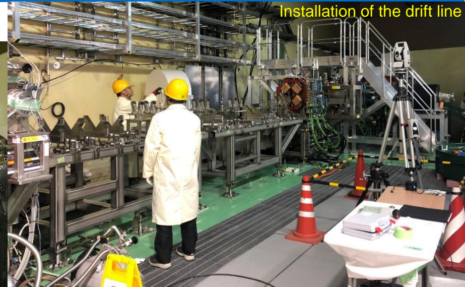
Connection of the vacuum components in a portable clean booth
