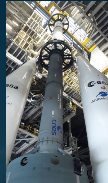
ECT Central Core Deployment and ESRs mating in Launch Zone (CCDZ)
