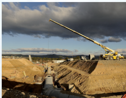
Site Adaptation Works: trenches
