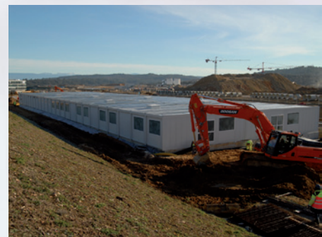
Site Adaptation Works: canteen
