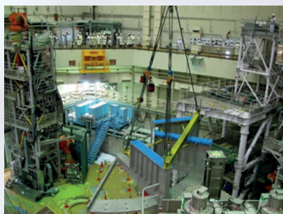
Assembly of Cryostat Base
